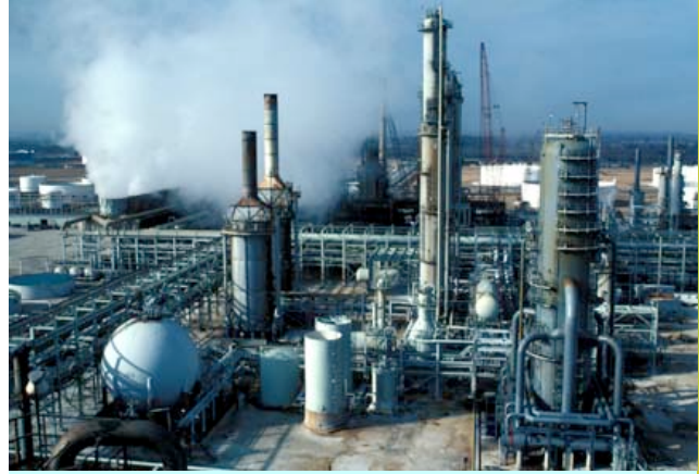
The process of turning oil into a usable fuel contributes to air pollution.
