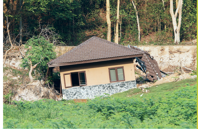
A house destroyed by a landslide
