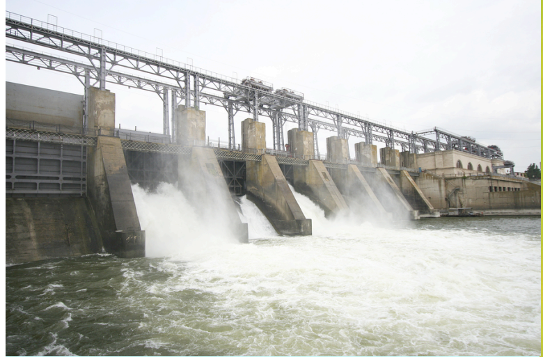
At a hydroelectric power plant, river water falls over a dam. The water turns turbines that generate electricity.
