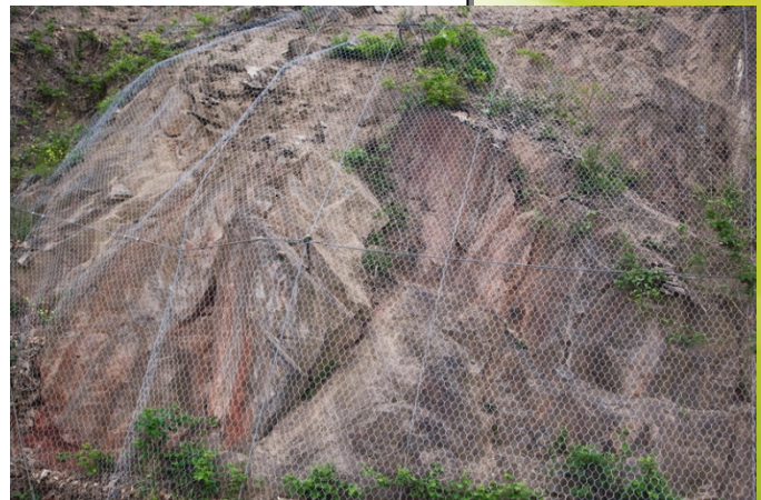
Putting a mesh net over loose rocks can help prevent the rocks from falling to lower ground and injuring people or damaging property.
