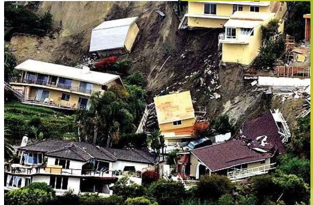
This damage resulted from a landslide near Laguna Beach, California, in 2005.
