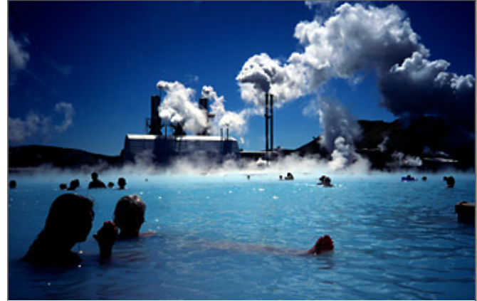
Icelanders relax in a hot spring while a geothermal power plant produces electricity.
